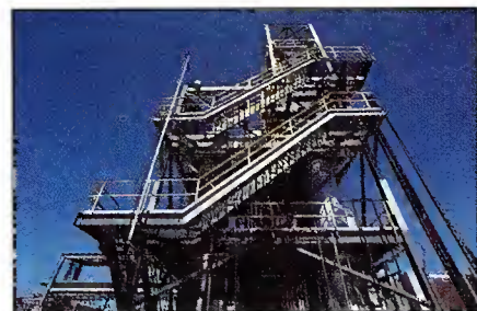
A solvent recovery tower at a magnetic tape plant. State-of-the-art facilities, such as this, now recover nearly 95% of all reclaimable raw materials. (Courtesy of Ampex.)
